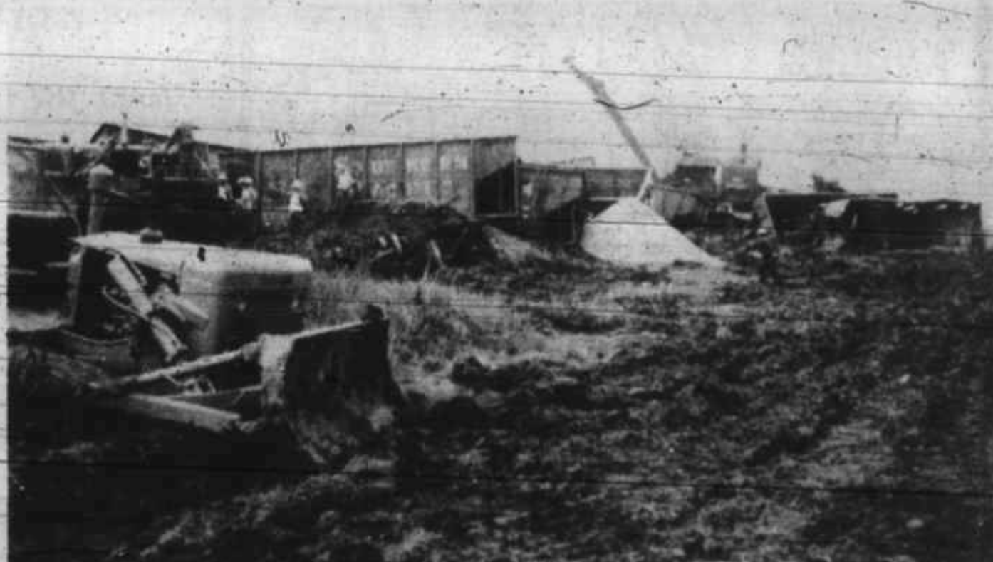
Southern Pacific crewmen are shown untangling the huge pile of steel and sand and gravel at the site of the 23-car derailment on the Bellaire Branch, six miles southeast of
